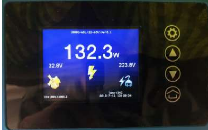
Main „Power View“ display during normal operation
